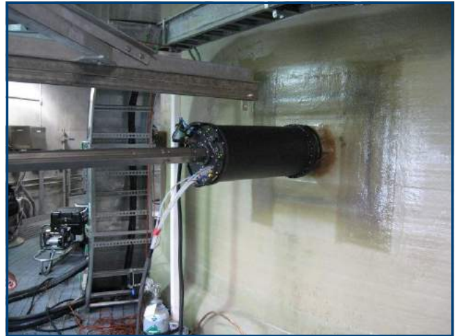
PPU standard configuration for stack flow test
